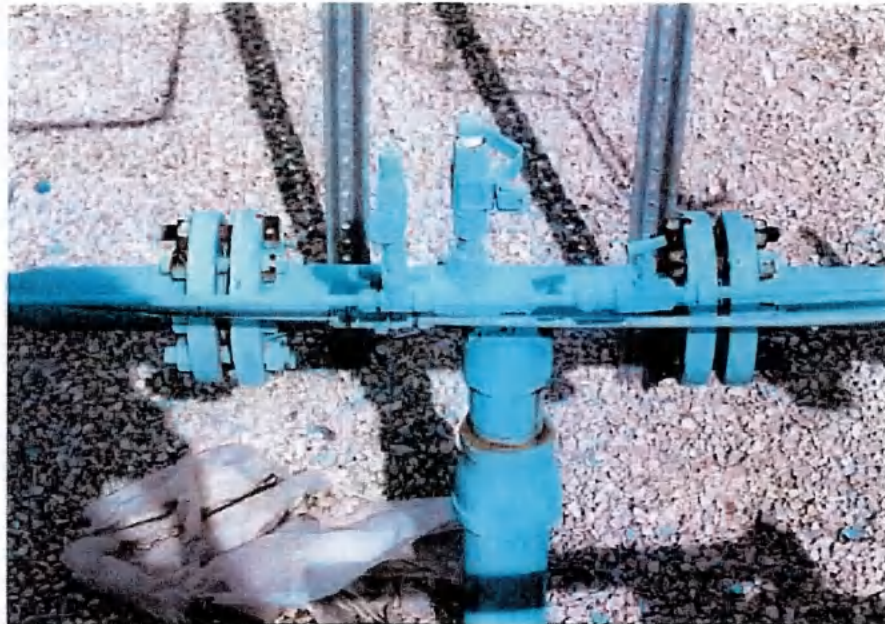
Photograph 3 – Example of piping within limits of Good atmospheric condition
